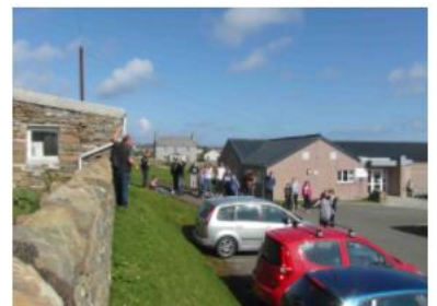
Installing another camera (Westray I think!)
